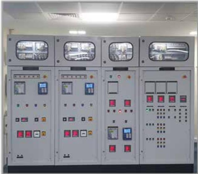
Fig. 3.76: Control System for Power Testbed
